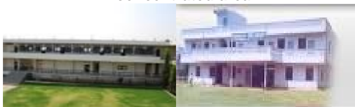
Figure-4.1: Construction of Primary Schools under SSA in minority concentrated area
